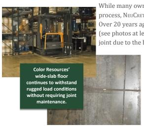
While many owners, developers and engineers consider wide-slab construction a new process, NeuCrete has been developing and perfecting steel fiber technology for decades. Over 20 years ago we first designed a floor for Color Resources utilizing fiber technology (see photos at left) and today that floor is still in operation and has only one crack, a cold-joint due to the batch plant breaking down. During that same time we designed a 700,000
